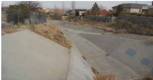
ENGINEERED STORMWATER CHANNEL
